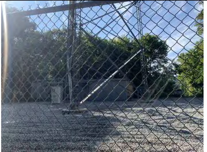
6. View of the existing compound, view to the northwest.
