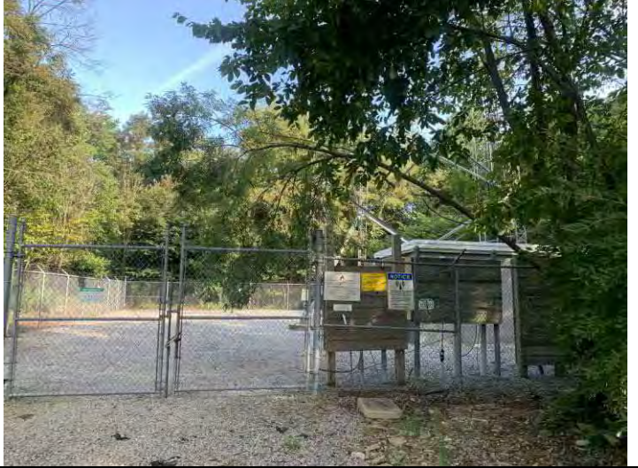
2. View of the existing compound, view to the southeast.
