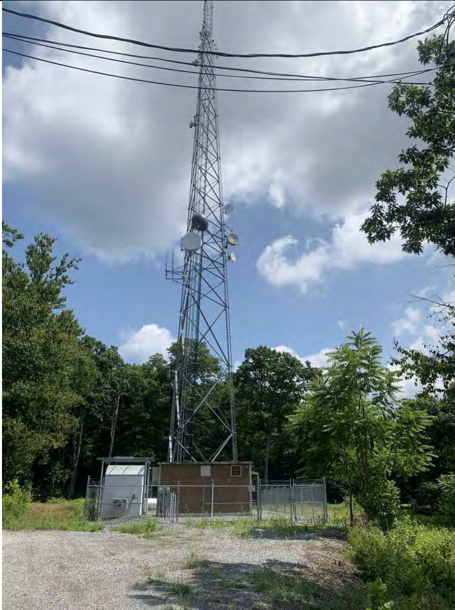
11. Overview of the existing tower compound, view to the northeast.
