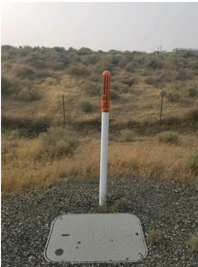
Photo 4: Constructed handhole/vault.
