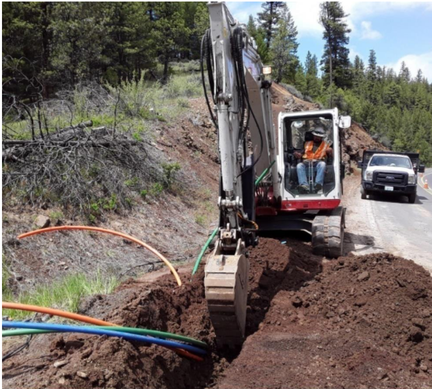
Photo 2: Fiber-optic conduit placement via trenching method (photo credit: Zayo Group, LLC).
