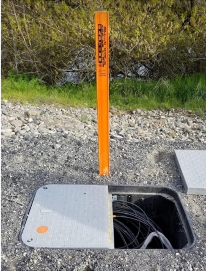
Photo 11: Marker for line-of-site and vault locations.
