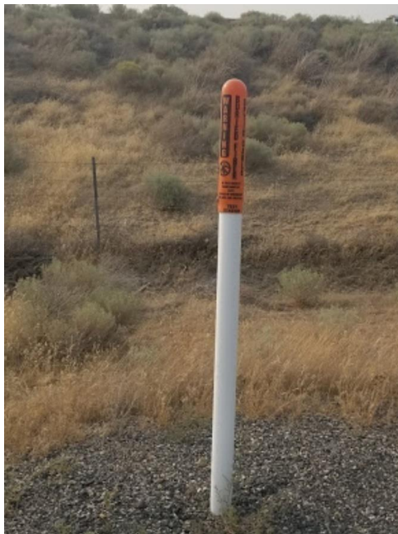
Photo 10: Marker at splice points.
