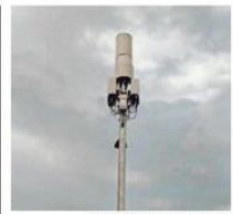
SDN COMMUNICATIONS/SUBMITTED A "small cell" cell tower atop a light pole stands as an example of technology being rolled out by Verizon Wireless and others, seeking to add capacity to the mobile data network and prepare for the next generation of high-speed mobile broadband.
